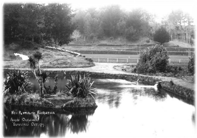
View of Eastern Terraces 1897. Those terraces were not properly developed until 1907.
