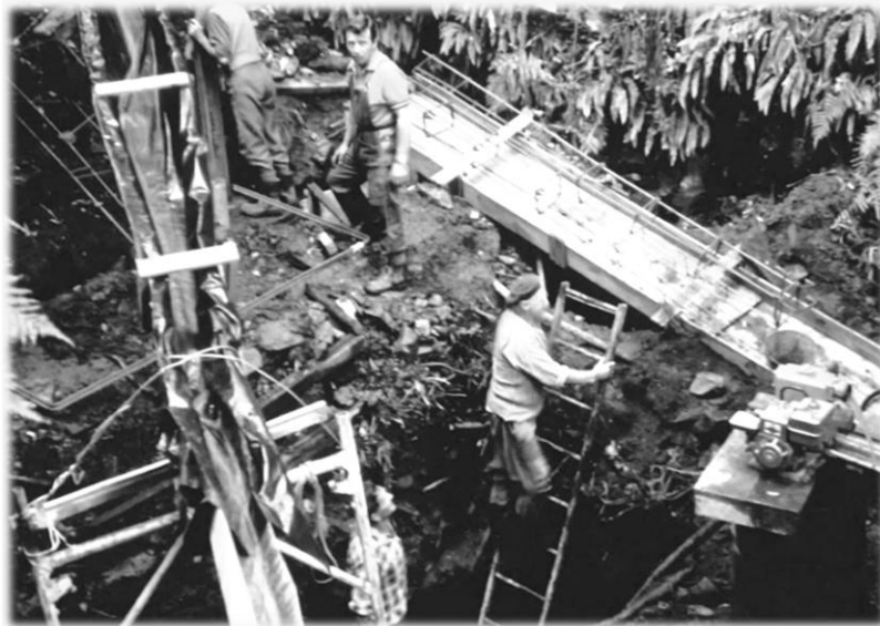
In search of solid ground for foundations.
