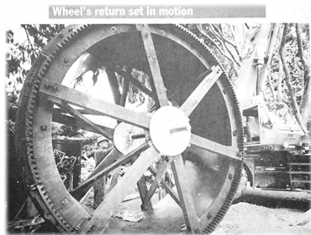
New Waterwheel ready to be installed. TDN , Nov 1, 2005.
