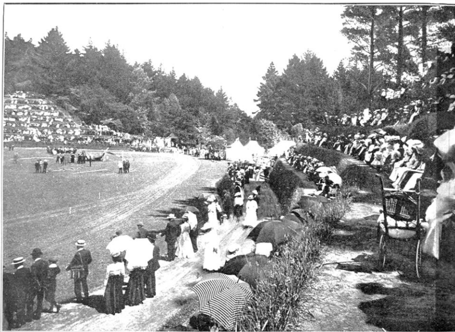
Opening of the new Sports Ground. AWN , Jan 16, 1908.
