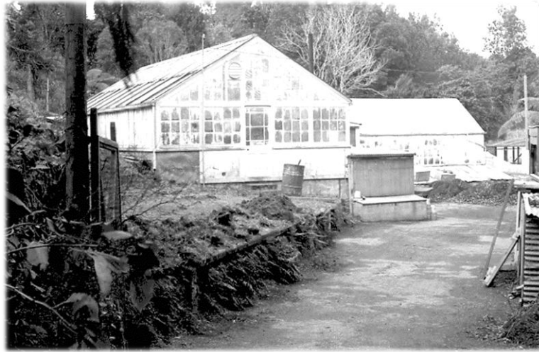
The two glass houses moved from Brooklands in the late 1930s. The begonia house in the foreground, the propagating house behind. Collection of Puke Ariki (Ref: ARC2011-029).
