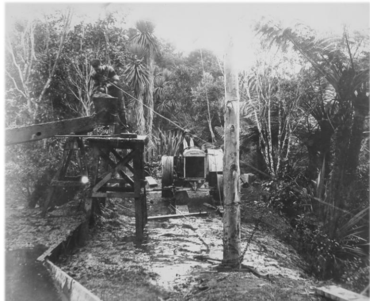
Park tractor winching buckets of silt from the lake. Collection of Puke Ariki (Ref: A.4.18).
