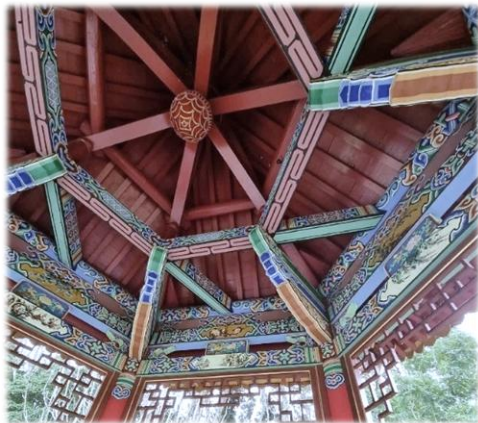
Spring Wind Pavilion. Freestyle Hand Painted Roof.
