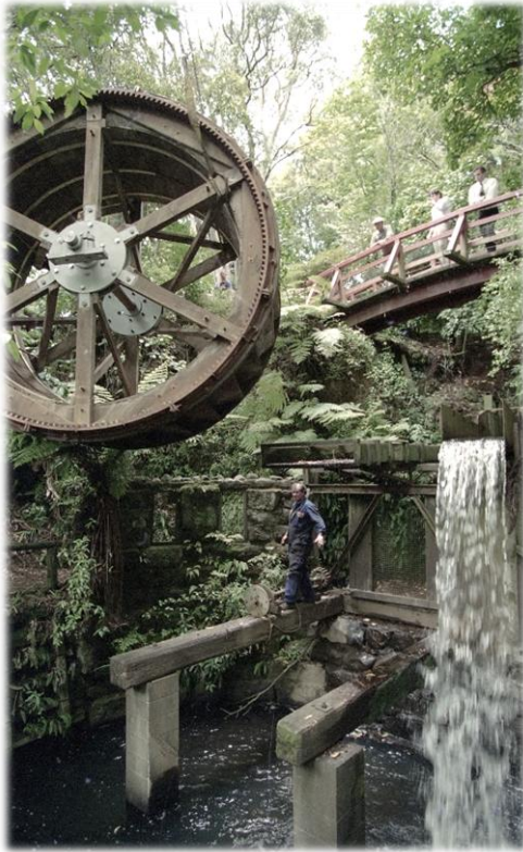
Waterwheel being lowered into position. TDN , December 10, 1993.
