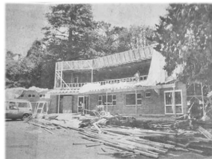
1988 Extension under construction. TH , December 12, 1988.
